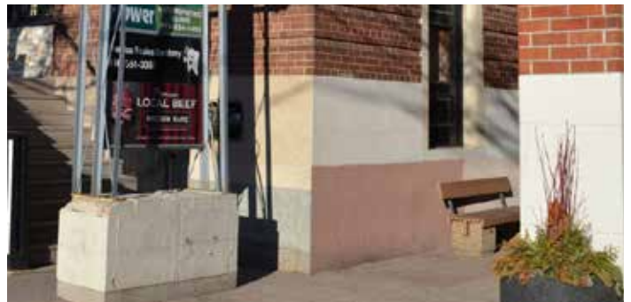
Figure 28: Typical conditions of the east elevation foundations, EVOQ
