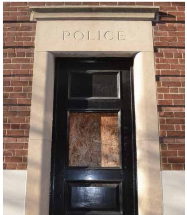
Figure 7: Secondary entrance of the Georgian Revival volume, EVOQ
