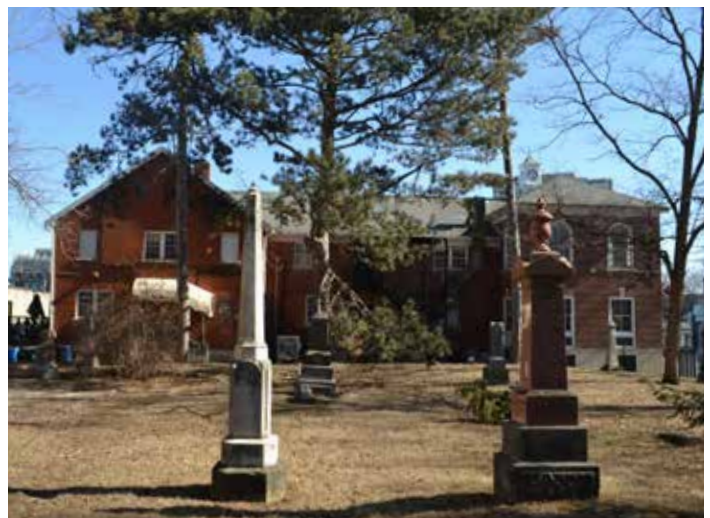
Figure 5: View of the Subject Property looking east, EVOQ
