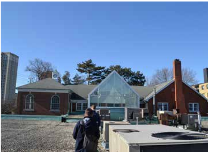
Figure 37: General view of the historic building's roof, EVOQ
