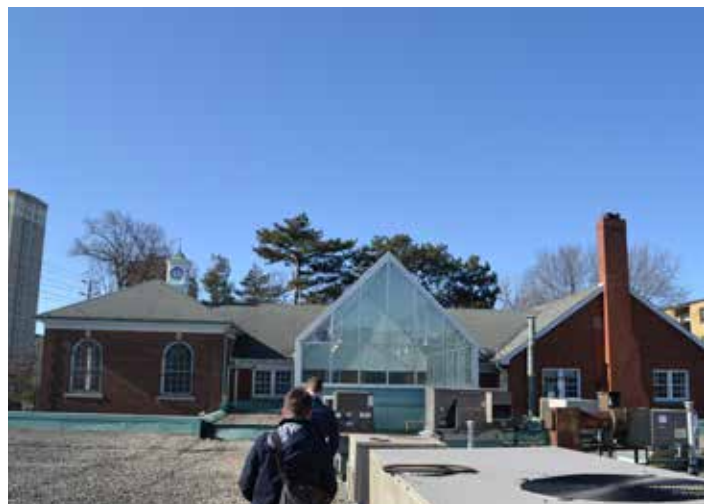
Figure 9: Skylight attachment to the original church volume, EVOQ
