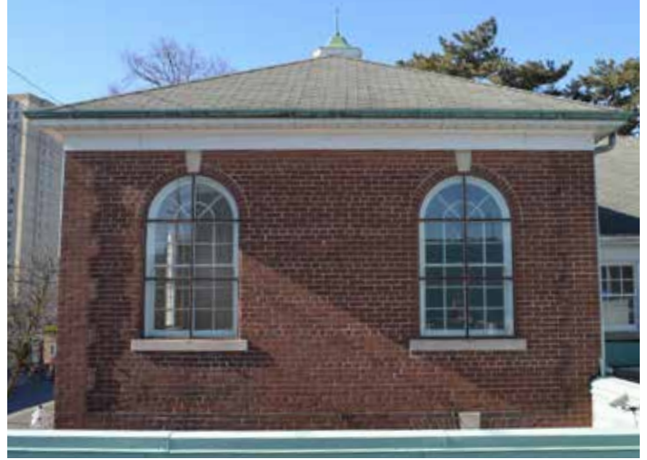
Figure 33: Windows on the west elevation with storm windows, EVOQ
