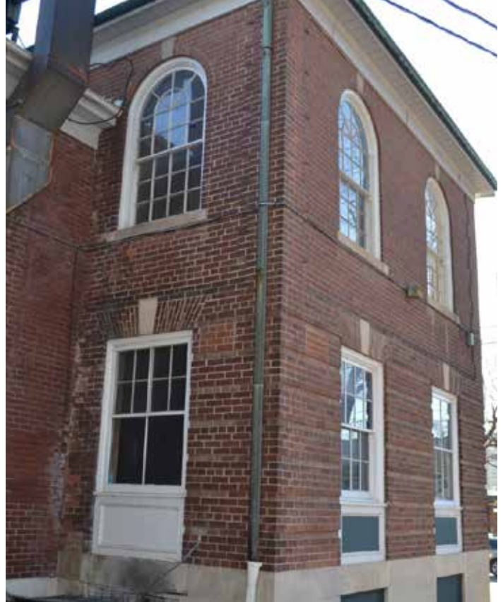
Figure 34: Typical window conditions of the 1940s addition, EVOQ
