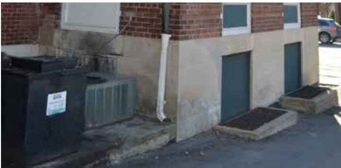
Figure 27: Typical conditions of the west elevation foundations, EVOQ
